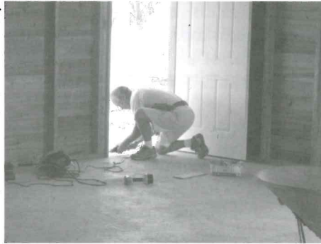
Robichaud helps to make the school building take shape
