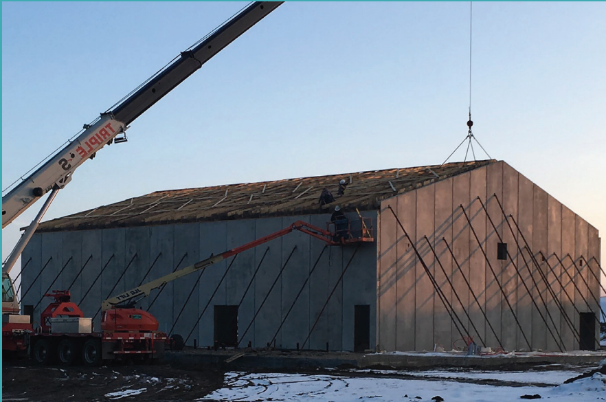
Gym walls and trusses now in place!
