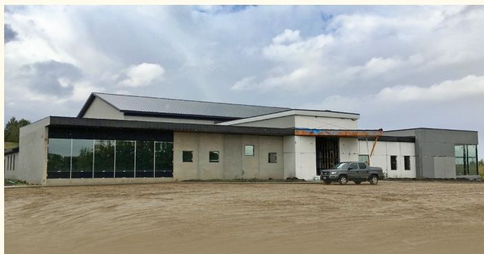
Construction of the high school continues to progress.
