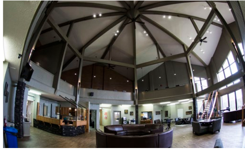
Renovation of Lakeview Hall's lobby.
