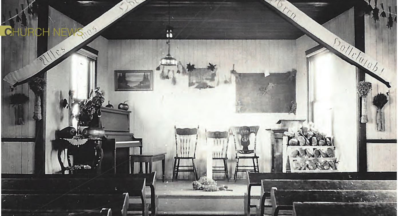
A rostrum on the south end of the church, added circa 1928, was used for preaching the Word, in addition to numerous MV (Missionary Volunteer) meetings or youth meetings and special event gatherings. During the winter time, the gas lanterns were pumped up as members returned to the church after completing their chores to fellowship together for the evening. Music, recited poetry (not read), and special features were a highlight enjoyed by all. Participation was a privilege. Everyone wanted a part! Depicted here is a typical Thanksgiving celebration. The banner translation is something similar to "In everything give thanks to the Lord. Halleluiah!"
